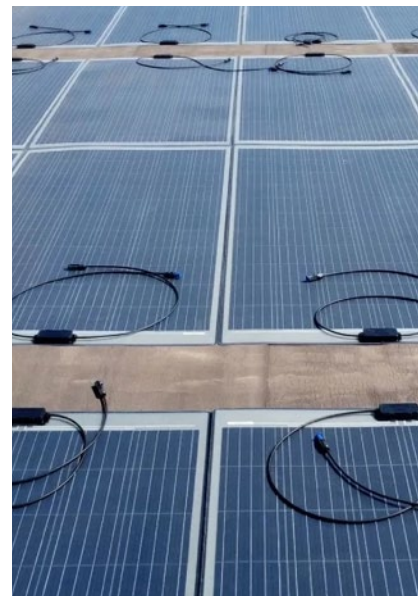
DAS Energy modules installed on bitumen
