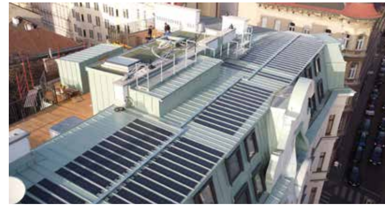
metal sheet roof / privat
