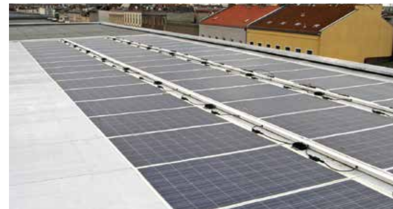
Membrane roof / Berlin
