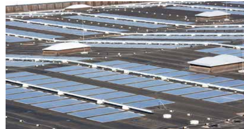
Bitumen Roof / Vöslauer Mineralwater
