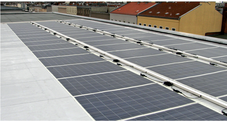
Membrane roof / Berlin
