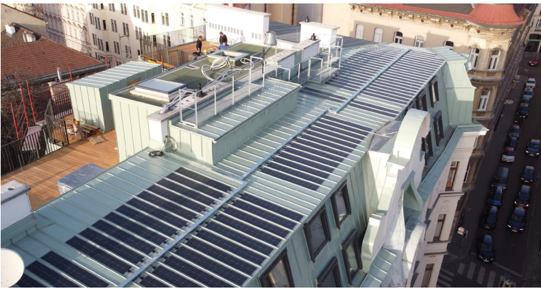
metal sheet roof / privat
