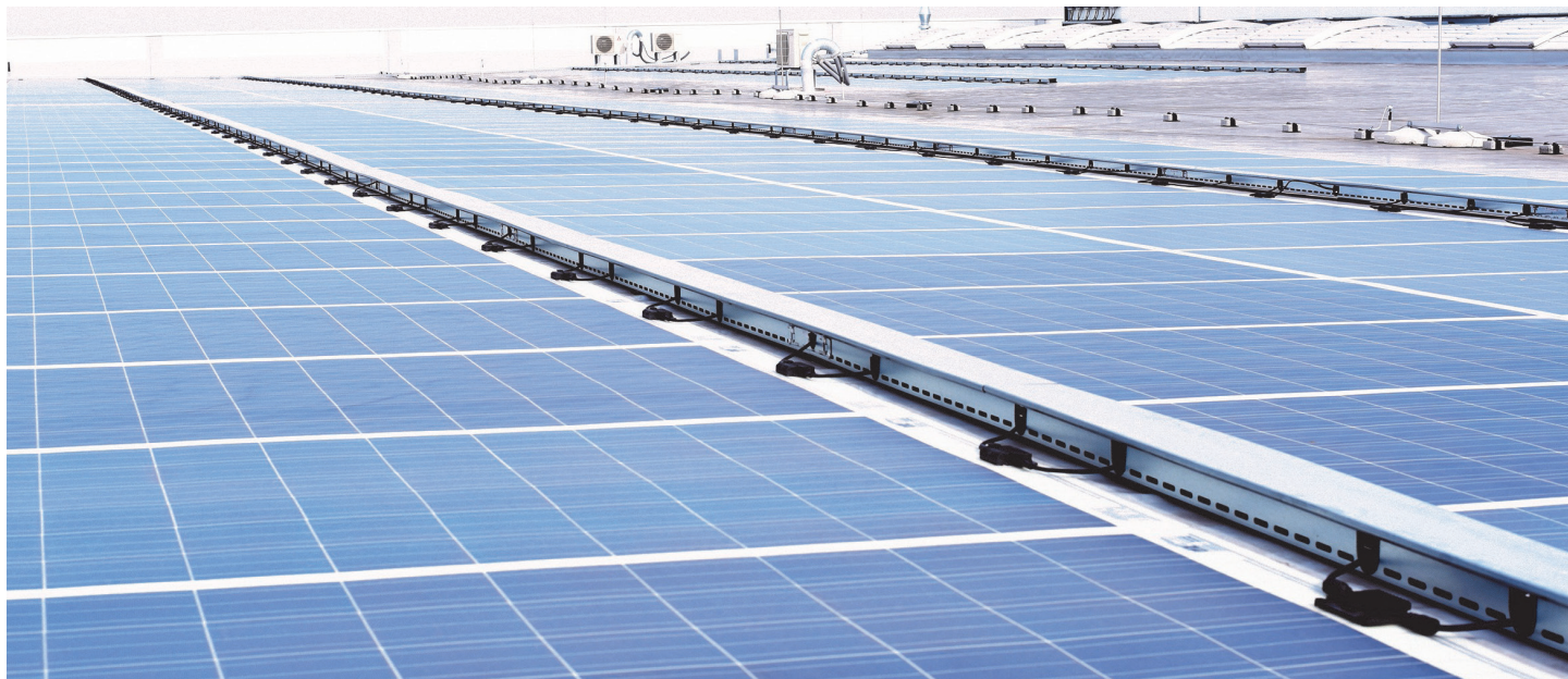
Rooftop installation DAS Energy Headquarters
