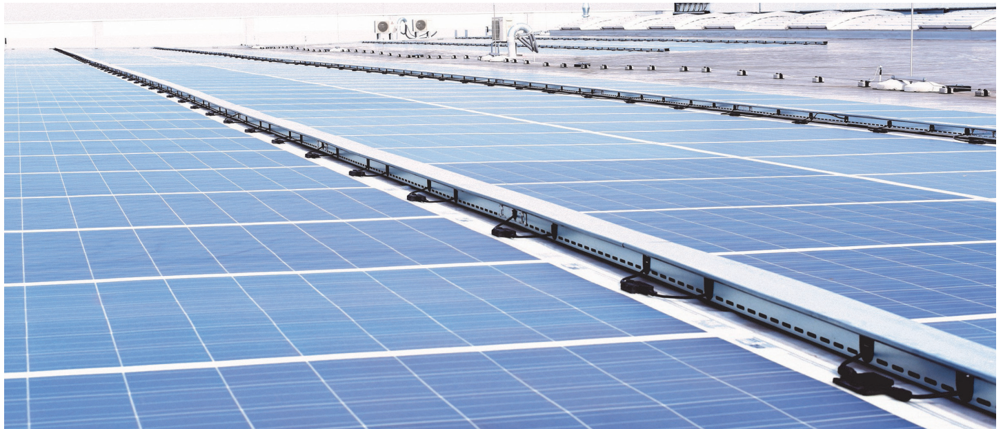
Rooftop installation DAS Energy Headquarters
