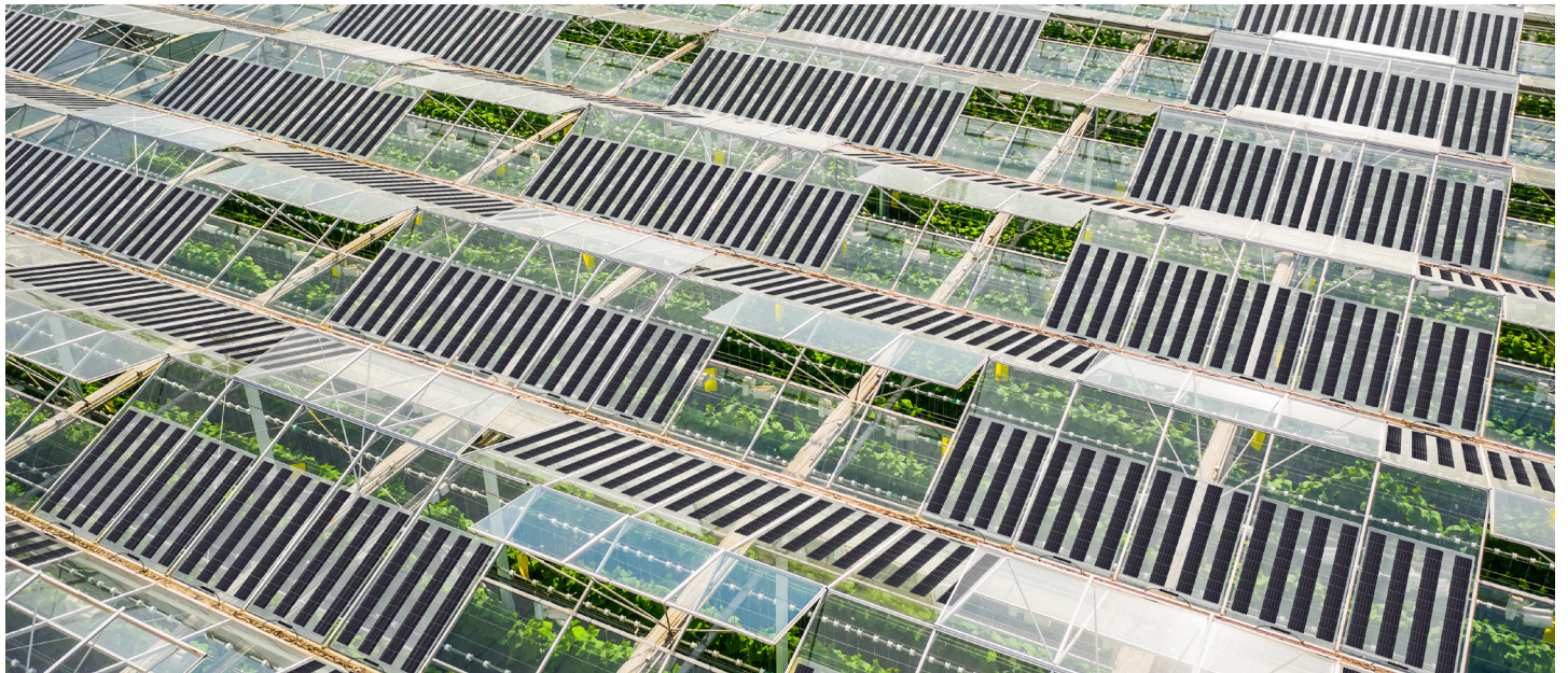
Rooftop PV installation / Greenhouse
