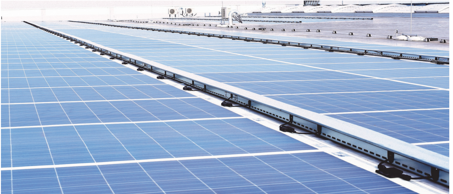
Rooftop installation DAS Energy Headquarters
