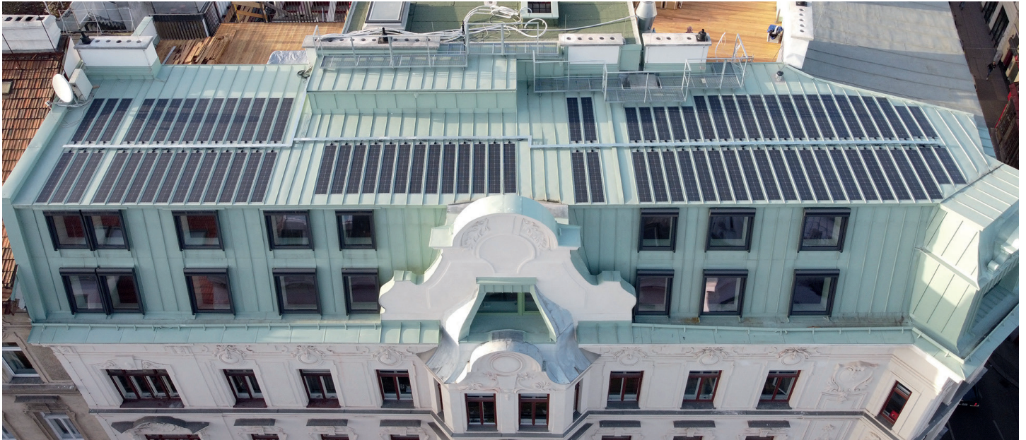
Rooftop installation private top floor, Vienna
