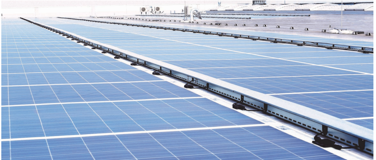
Rooftop installation DAS Energy Headquarters
